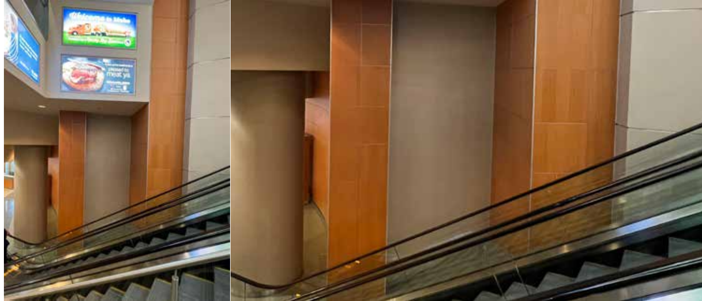
Boise Airport escalator from second to first floor, photo courtesy of Arts & History
