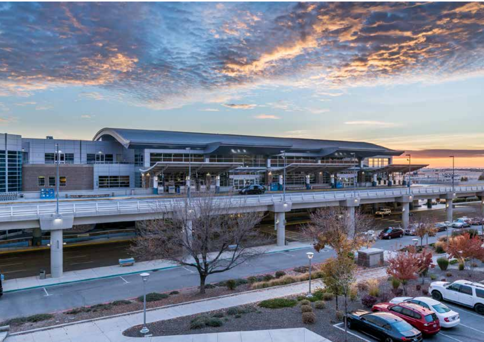
Boise Airport (2020), photo courtesy of Tory Taglio Photography
