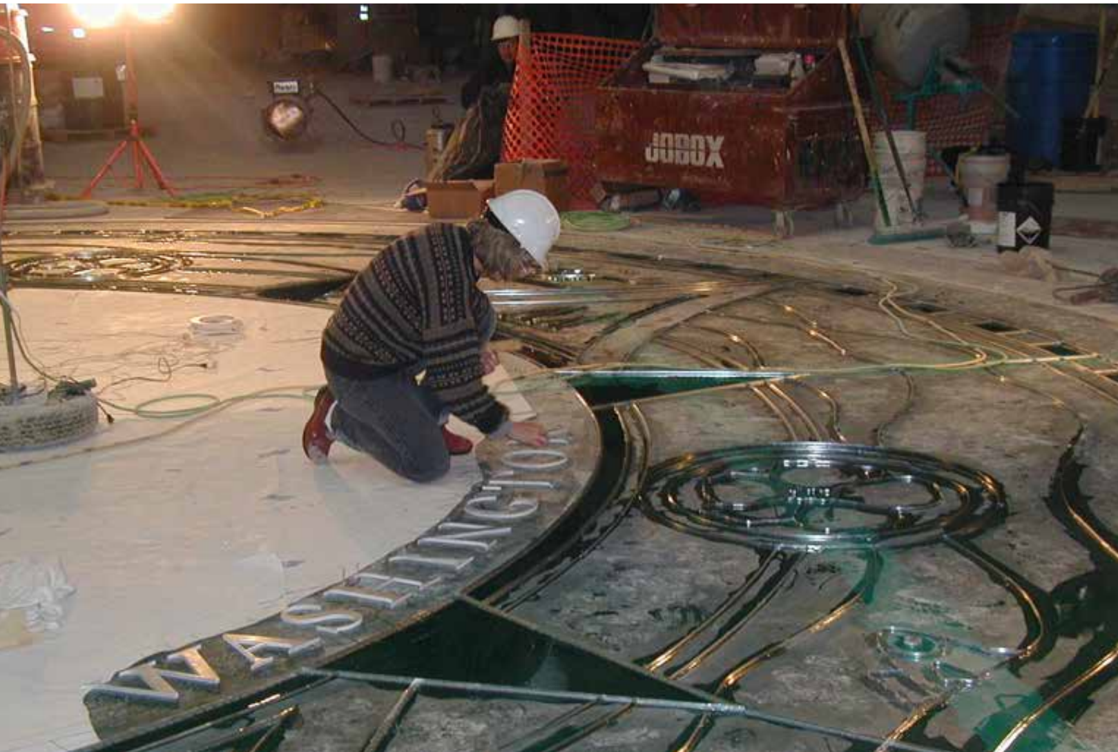
Terra Firma (2003) by Elizabeth Wolf, photo courtesy of Arts & History Elizabeth Wolf placing metal letters in the terrazzo floor.
