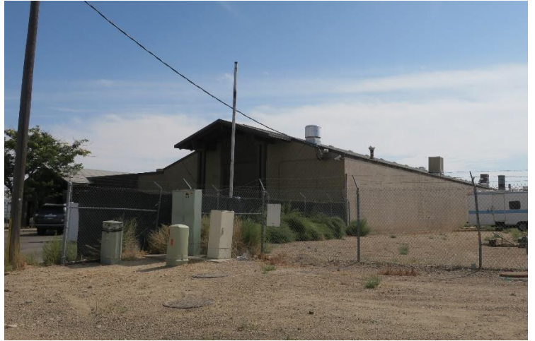
House of Hounds Building (037; BOI-17), view SE, April 2018
