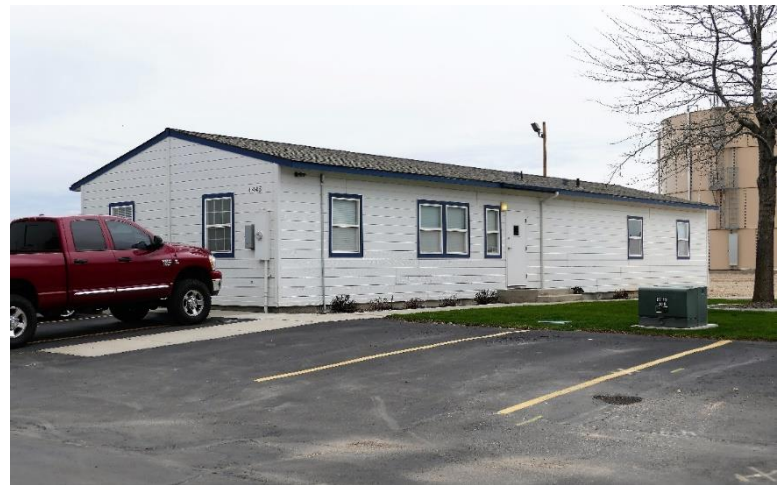
Modular Building (085; BOI-11), view SE, April 2018
