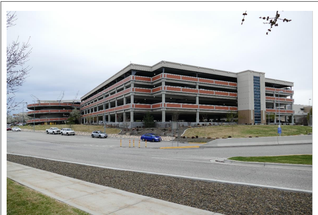
Boise Airport Parking Garage (014), view E-SE, April 2018
