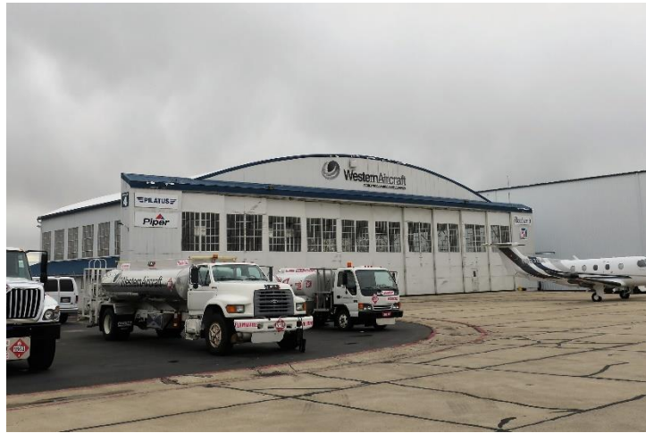
Large Single-Bay Hangar (080; BOI-06), view SW, April 2018
