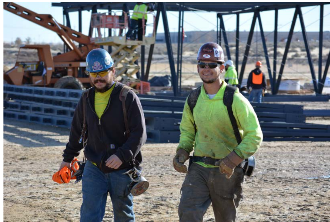
SkyWest Maintenance Hangar Construction, 2014
