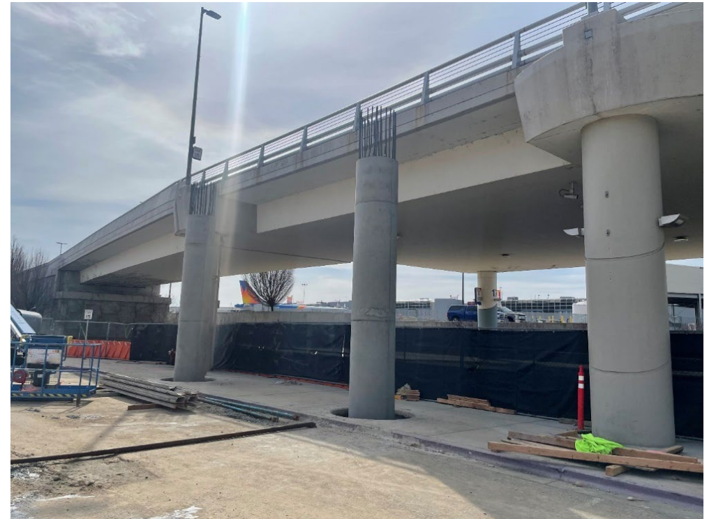
Pedestrian bridge piers
