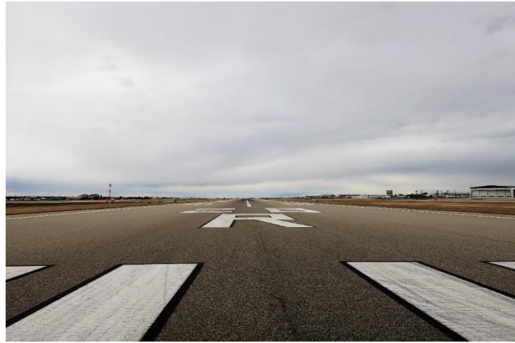
Runway 10L-28R (049), view NW, April 2018
