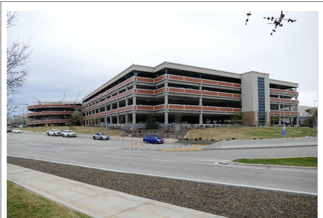
Boise Airport Parking Garage (014), view E-SE, April 2018
