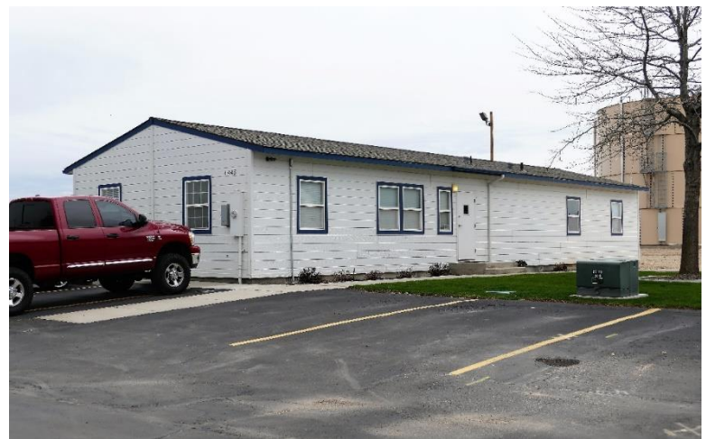
Modular Building (085; BOI-11), view SE, April 2018
